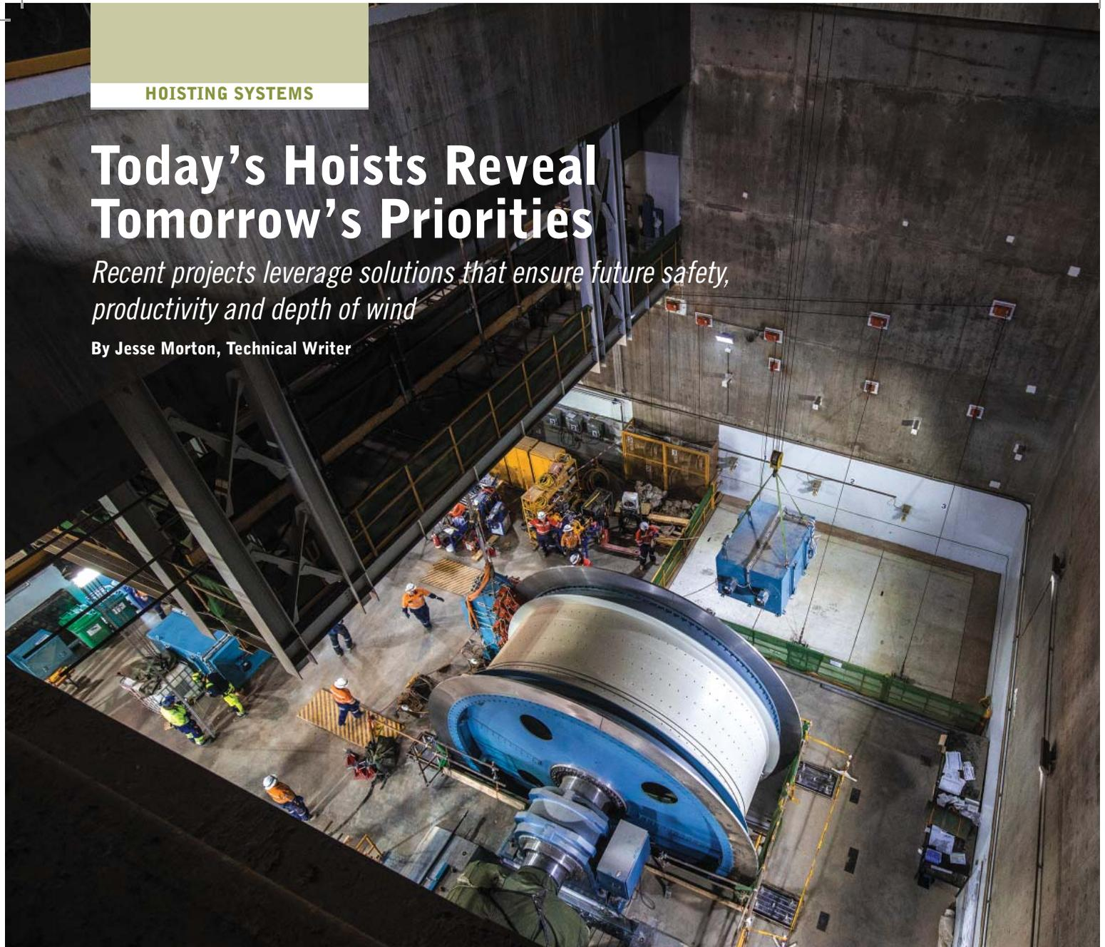
An overhead crane moves equipment and parts during installation of possibly the largest production friction hoist in the world, at Oyu Tolgoi. (Photo: The Redpath Group)
