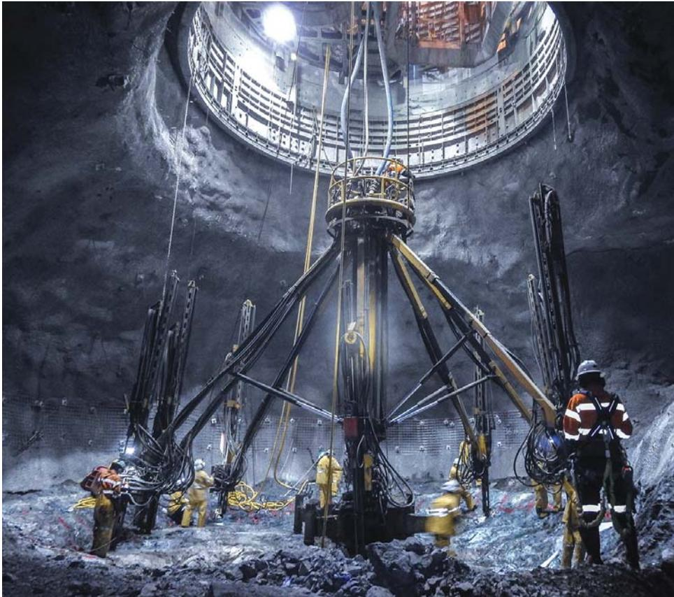
An 8-boom jumbo drill penetrates rock in the bottom of the developing No. 2 shaft at Oyu Tolgoi. (Photo: The Redpath Group)
