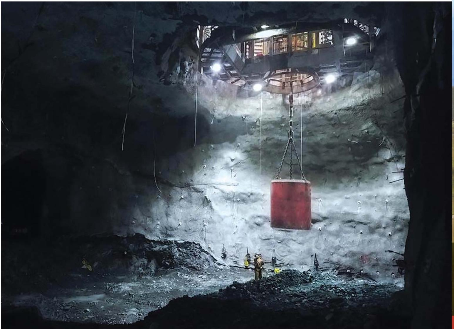
The Dayan Contract Mining team leveraged a three-stage Galloway during the sinking of the No. 2 shaft at Oyu Tolgoi. (Photo: The Redpath Group)
