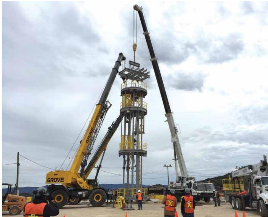
Two cranes are used to lower the Galloway into the shaft. (Photo: The Redpath Group)
