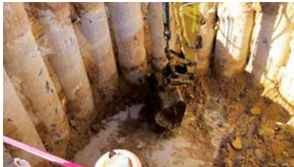
Clean up of the bottom of the excavated 4m deep hole.
