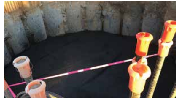
Centre of piles being filled with 12MPa blinding.
