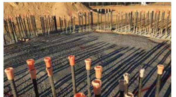
Completed and ready for raisebore pad.
